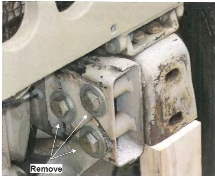
FIGURE 11. REMOVE EXISTING FRAME BOLTS
